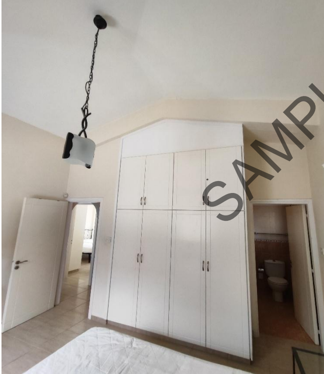
P3- The internal ceilings were found in sound condition.
