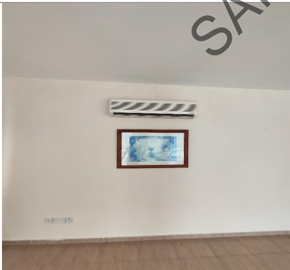
P1: Ac unit installation within the property.
