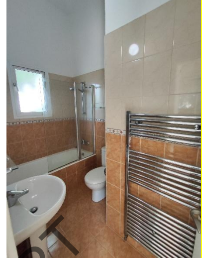
P3: Sanitary ware were found in sound condition.
