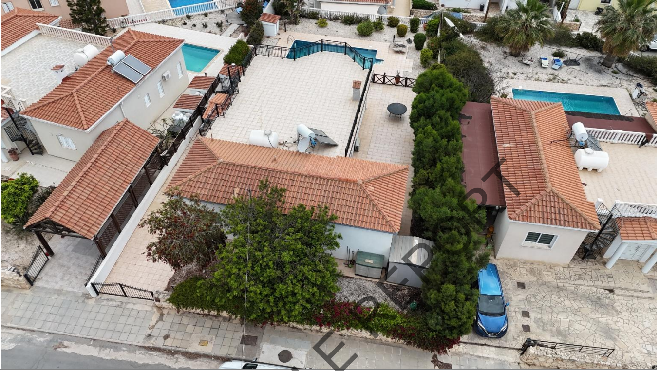
P1: External areas of the property at the time of the inspection.
