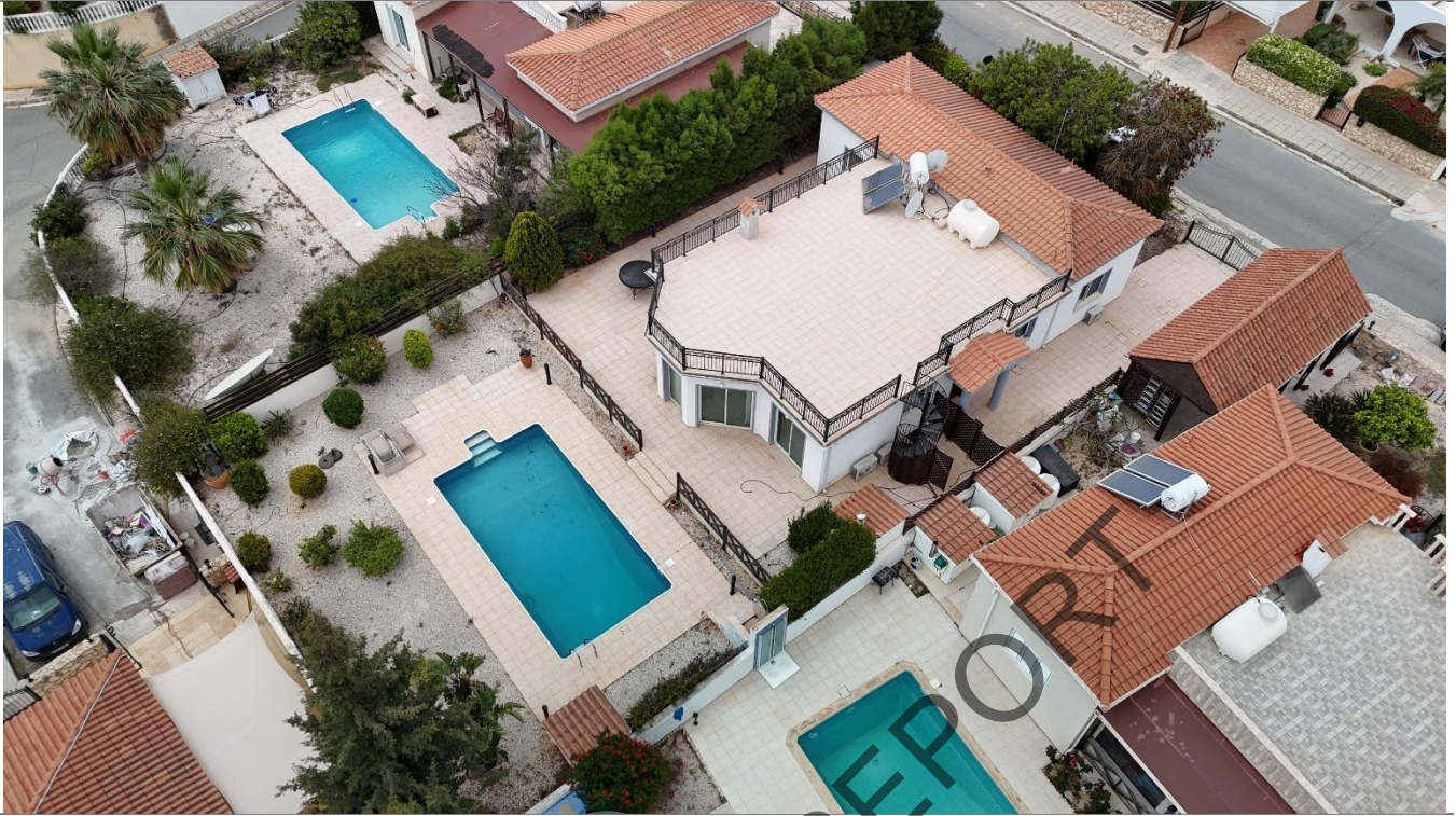
P3: External areas of the property at the time of the inspection.
