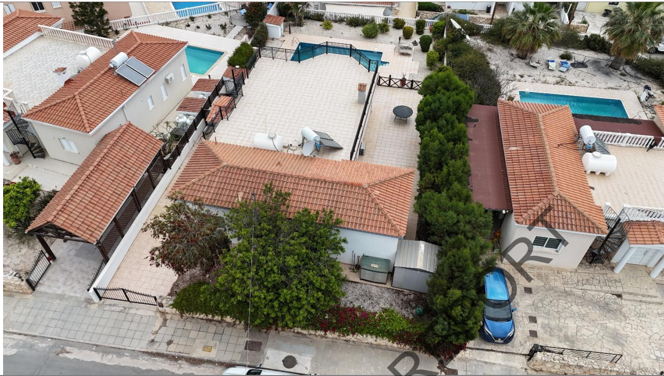
P1: The roof of the property was found in sound condition.
