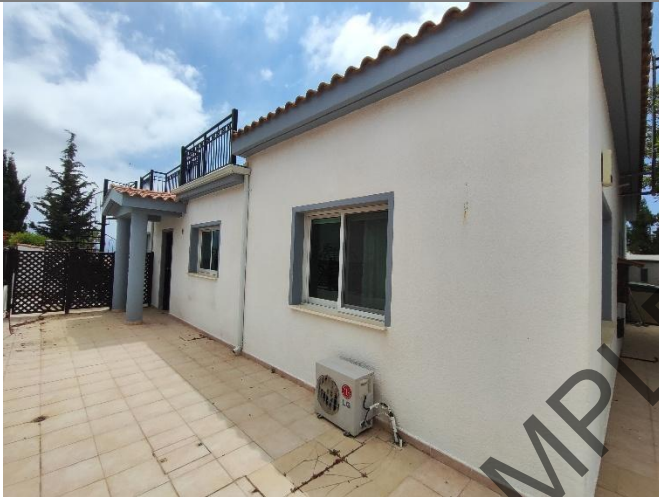
P3: External walls were found in sound condition.
