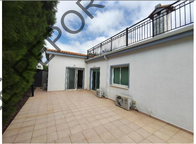
P4: External walls were found in sound condition.
