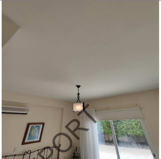
P2- The internal ceilings were found in sound condition.
