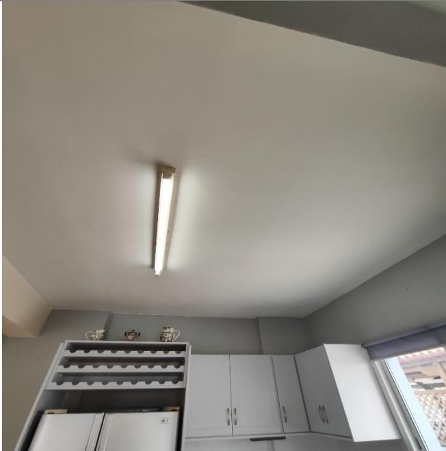
P1- The internal ceilings were found in sound condition.
