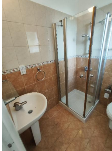
P2: Sanitary ware were found in sound condition.
